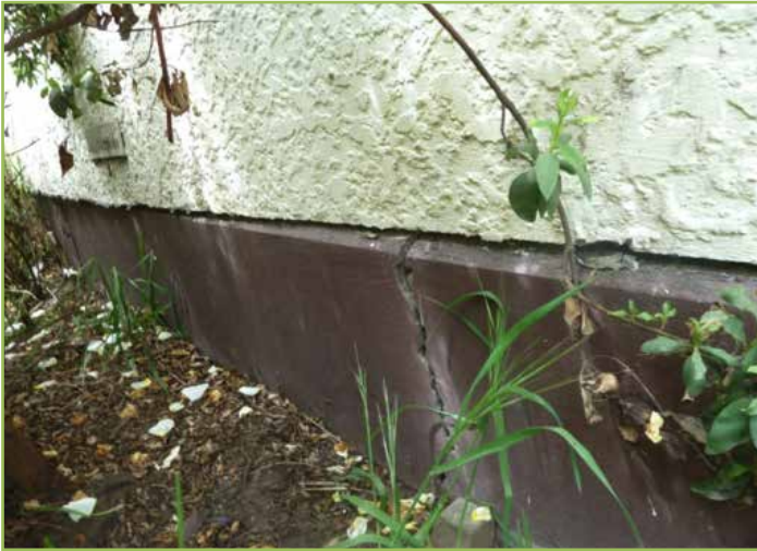
Foundation damage
