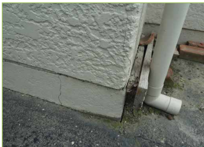
Foundation damage
