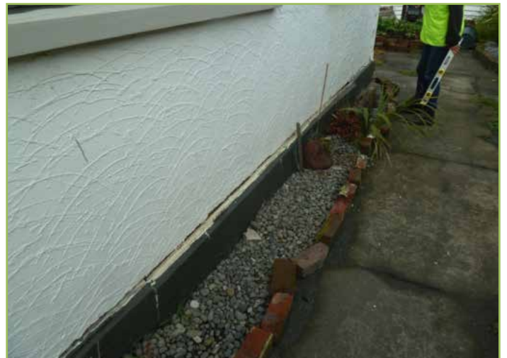
Foundation damage
