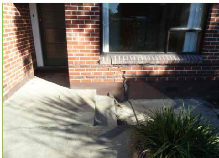
Foundation damage
