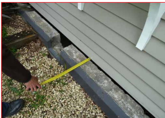
Foundation damage
