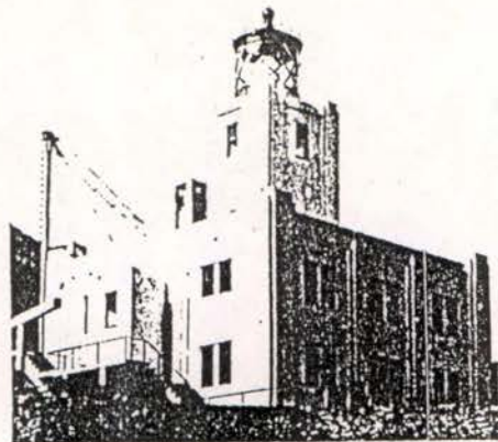
Figure 11-17. Scotch Cap Lighthouse on Unimak Island in the Aleutian Islands before the April 1, 1946, tsunami.
