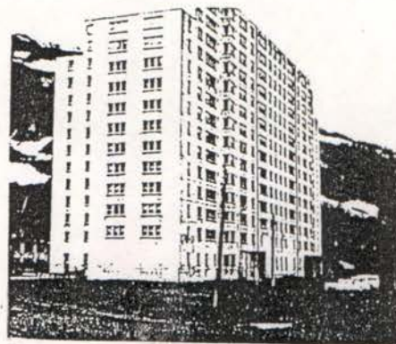
Figure 11-14. Hodge Building at Whittier, Alaska, after the 1964 earthquake. Building suffered between minimal and moderate structural damage.
