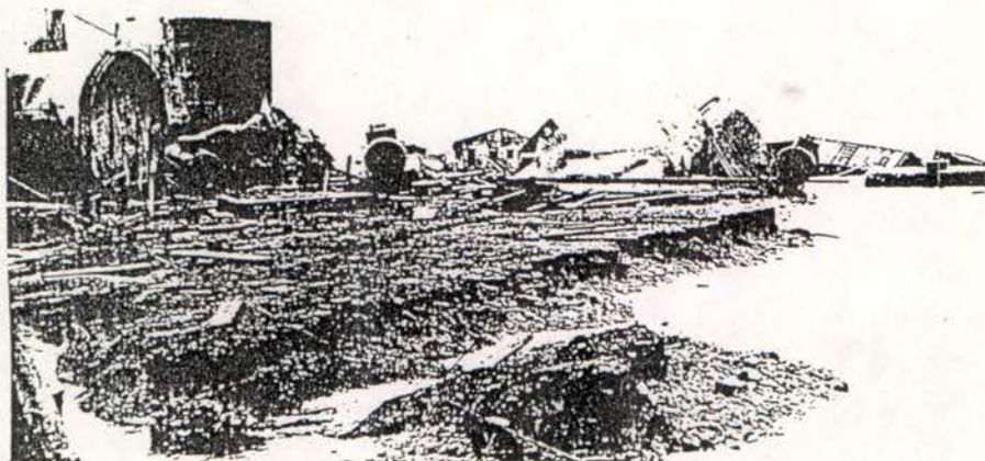
Figure 11-7. Texaco oil tanks after the 1964 tsunami and fire at Seward, Alaska.
