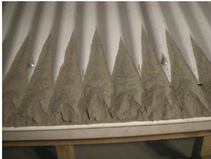
Fig. 12: Deposition of ash on a roof tilted at 45°. Talus-like aprons of ash accumulation once spouting is infilled. Position of ash within roof troughs remains static between 200 – 250mm from front edge of roof, with excess ash material shed over front lip of guttering.
