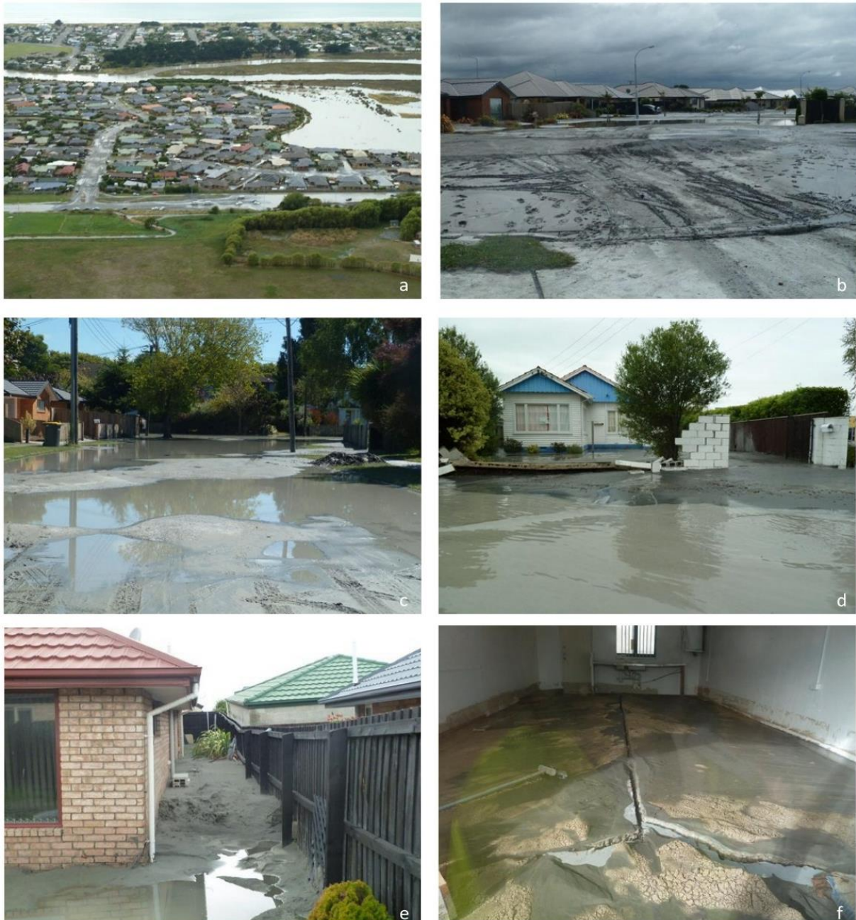
Figure 3.7: Observed liquefaction related land damage and residential house damage in Christchurch following the CES – reproduced from van Ballegooy et al. (2014b).
