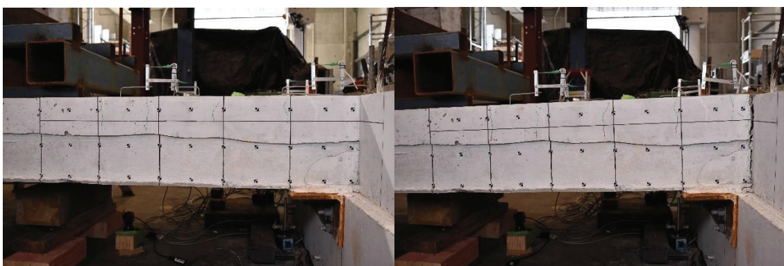
Figure 10: Specimen 2 Before Testing (Left) and at -2.75% Drift (Right)
