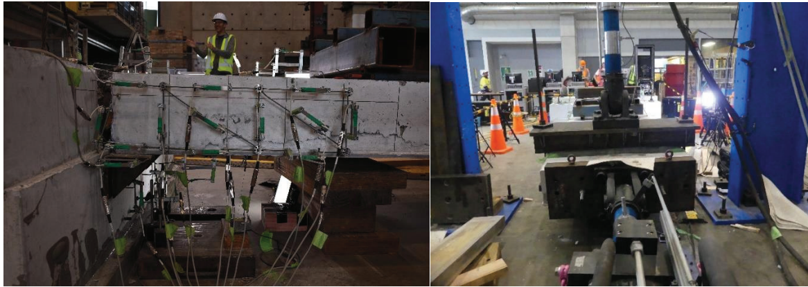
Figure 37: Specimen 6 - Out of Plane Twisting of Unit After Rupture of Two Starter Bars (-3.0% Drift)
