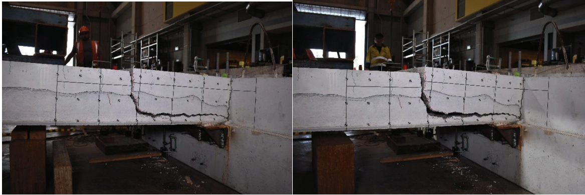
Figure 24: Positive 4.0% drift (Left) and Residual (Right) Showing Prying Effect of Separated Sections
