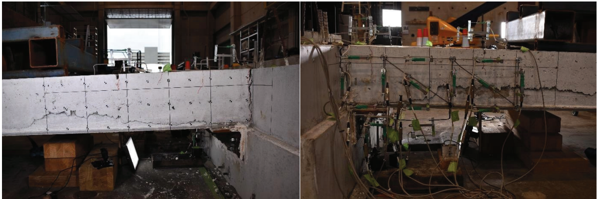
Figure 16: Specimen 3 at -3.5% Drift – All Damage Concentrated at Back Face (West – Left, East – Right)
