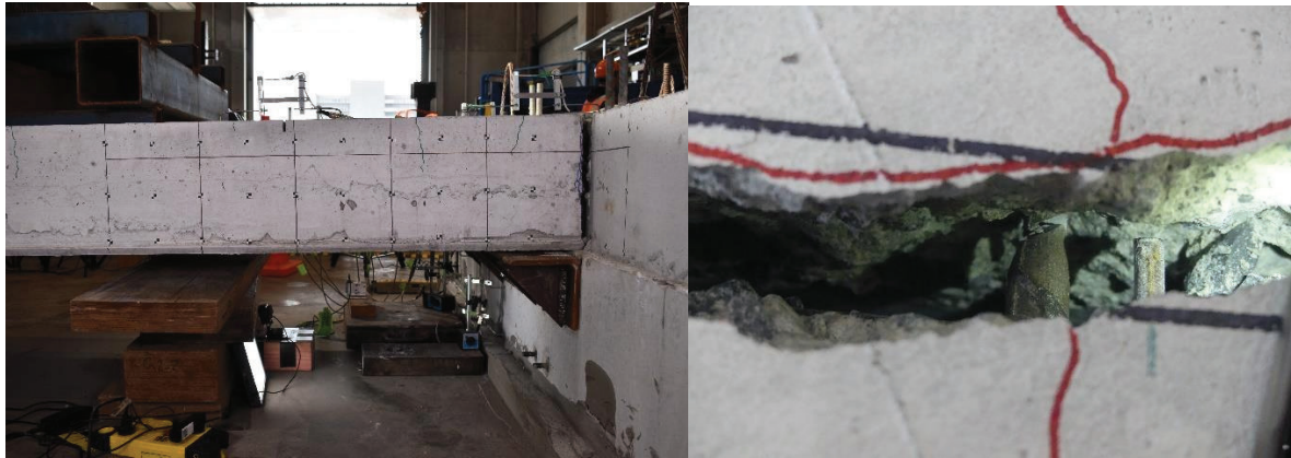
Figure 35: Specimen 6 at -2.0% Drift (Left) and Ruptured Middle Starter Bar (Right)
