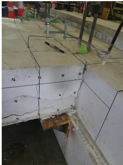
Figure 23: Full Depth Crack Propagation at Collapse
