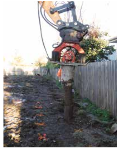
Above and below: Timber pole installation during the Ground Improvement Pilot Project, using a vibratory plate fixed to an excavator
