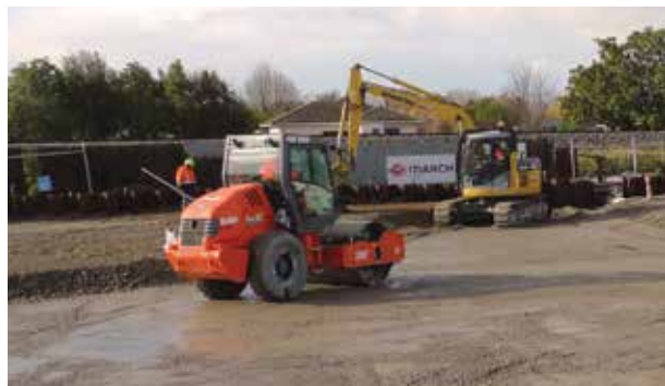
Roller compactor used to compact gravel
