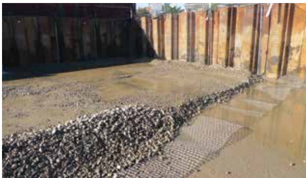
Reinforced gravel raft – geogrid and gravel installation
